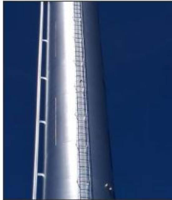
After Exterior coating renovations
