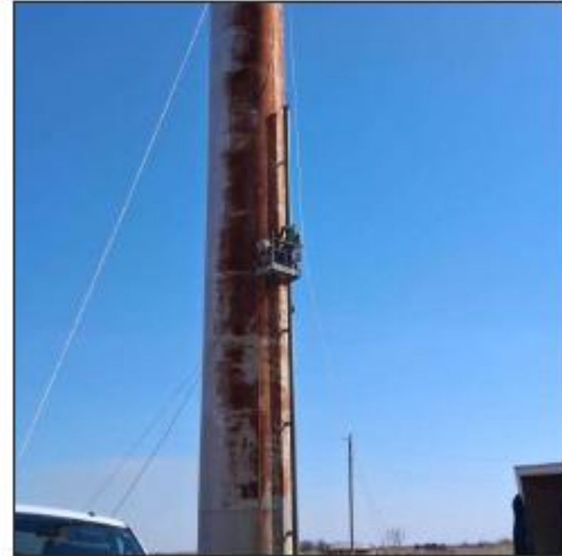
Before Exterior coating renovations
