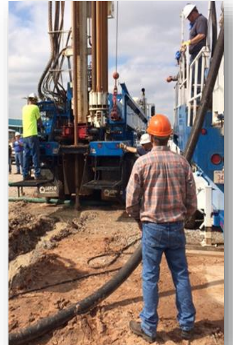
Training drillers to ensure proper well construction
